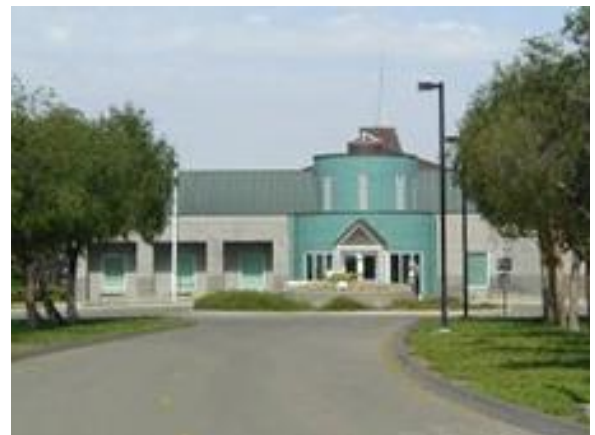
The Randall-Bold Water Treatment Plant is one example of a shared facility within the East Contra Costa County Region
