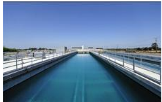
City of Brentwood Water Treatment Plant.
