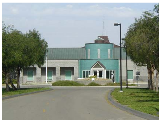
Randall-Bold Water Treatment Plant 40
